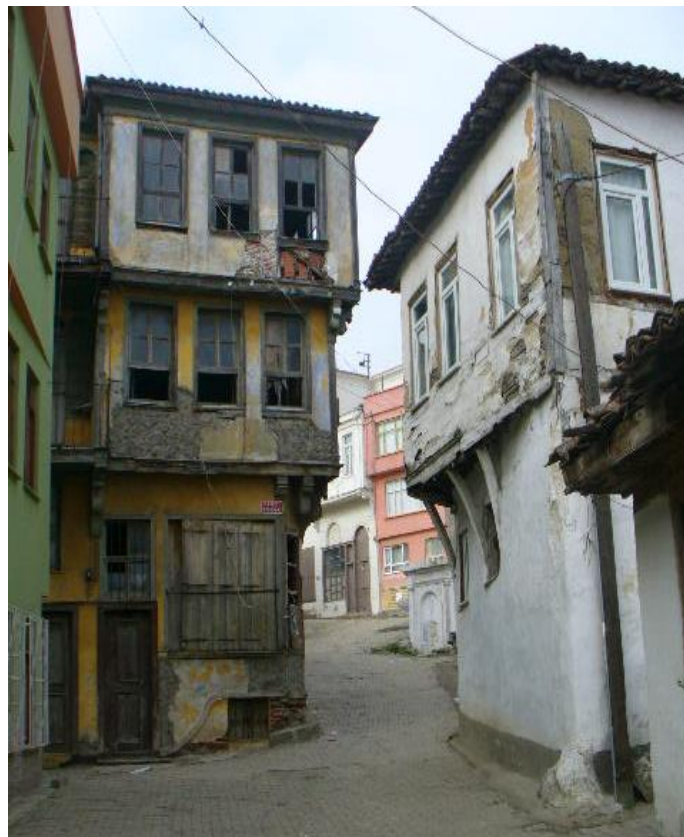
Figure 6. Two-three stories wood framed-masonry Trilye houses (P.A)
